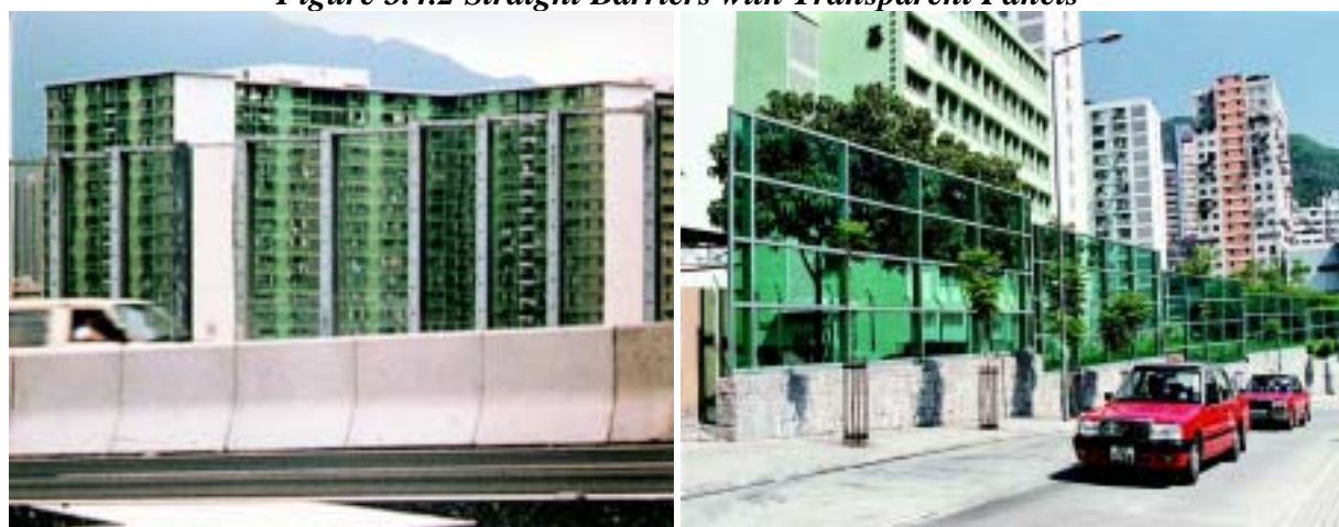
Figure 3.4.2 Straight Barriers with Transparent Panels
