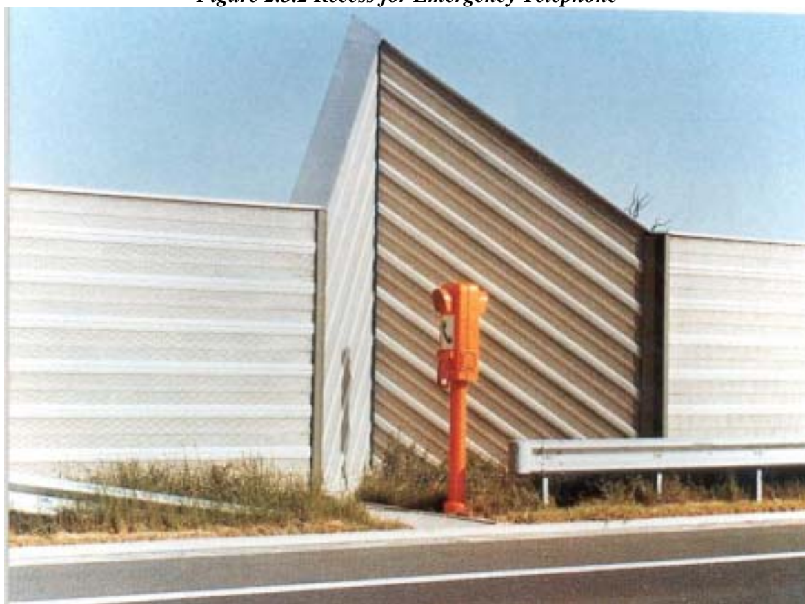
Figure 2.3.2 Recess for Emergency Telephone
