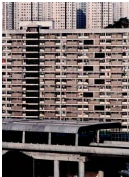
Figure 3.4.4 Transparent Panel in Semi-enclosure
